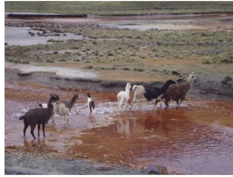
Figure 3: Leak of the dam at Milluni Chico – Llamas walking through and drinking the water
